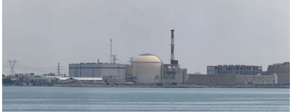
Bushehr nuclear power plant in Iran
