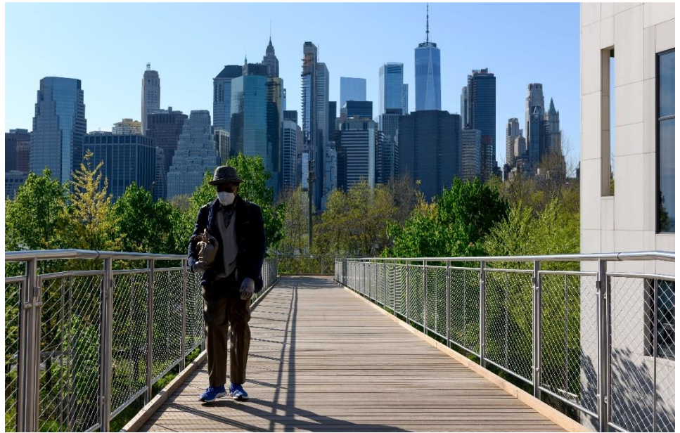
People walk on Brooklyn Bridge Park's rebuilt Squibb Bridge in New York.
