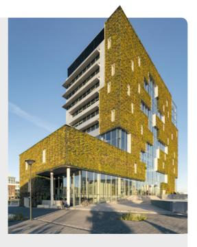
dismantled. There are several cycles in the building. The south façade is constructed using aluminium and is fully reusable without losing any of its value. The biological north façade consists largely of plants and greenery.
