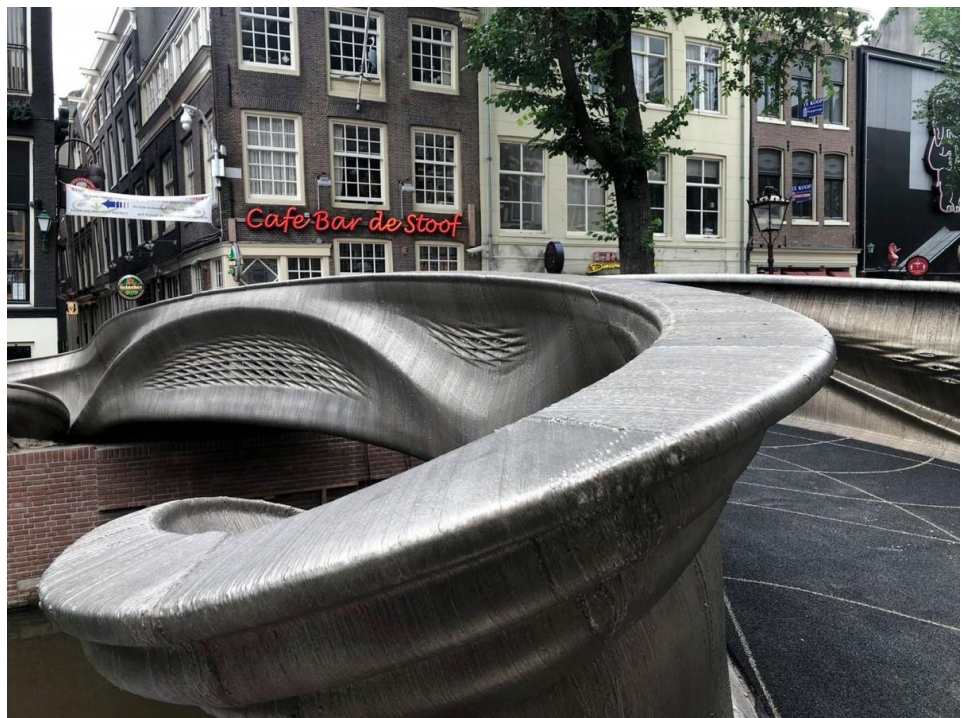
3D printed pedestrian bridge in Amsterdam shows that the technology is well-suited to making complex shapes
