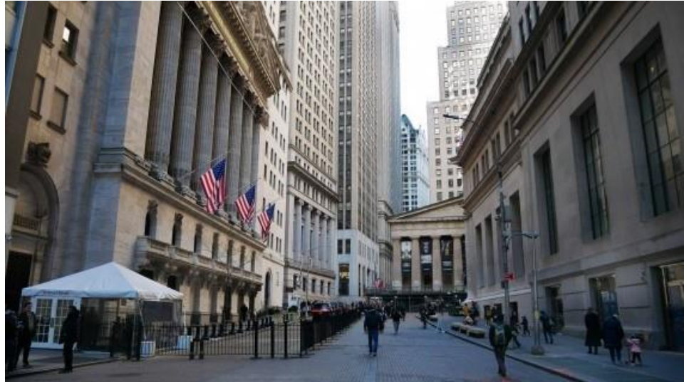
Wall Street, New York - March 2023
