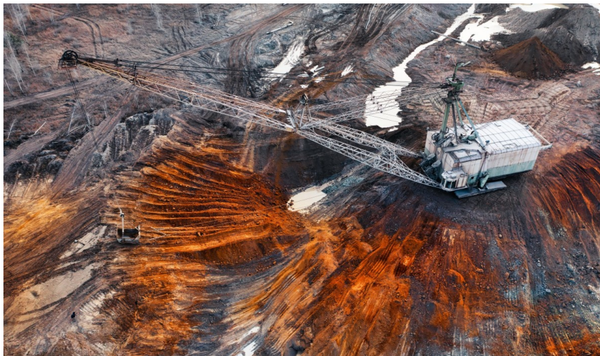
Where critical minerals begin: A walking excavator at work in a rare metals quarry
