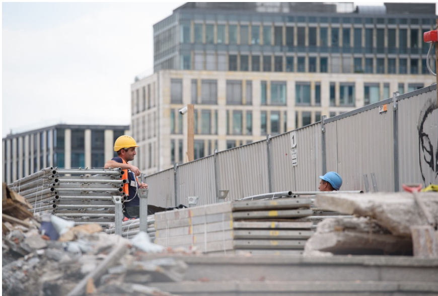
Construction work in Warsaw, Poland
