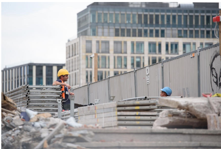
Construction work in Warsaw, Poland
