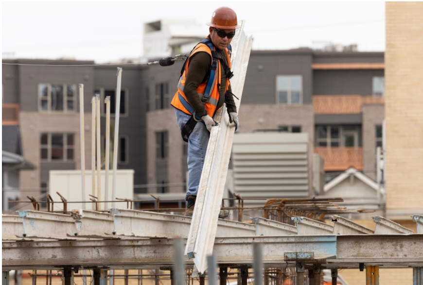
A construction worker in Washington DC
