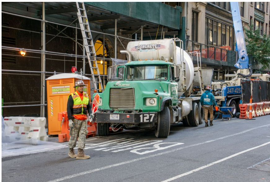
Workers at a construction site in New York
