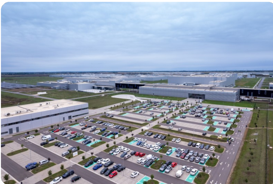
New BMW facilities in Debrecen are yet to move Hungary's industrial production numbers
