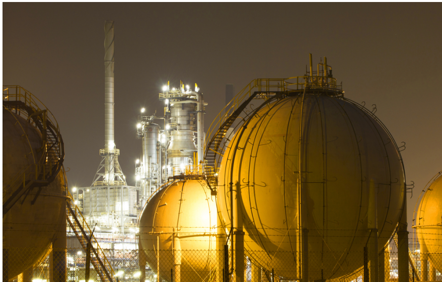
Gas storage tank
