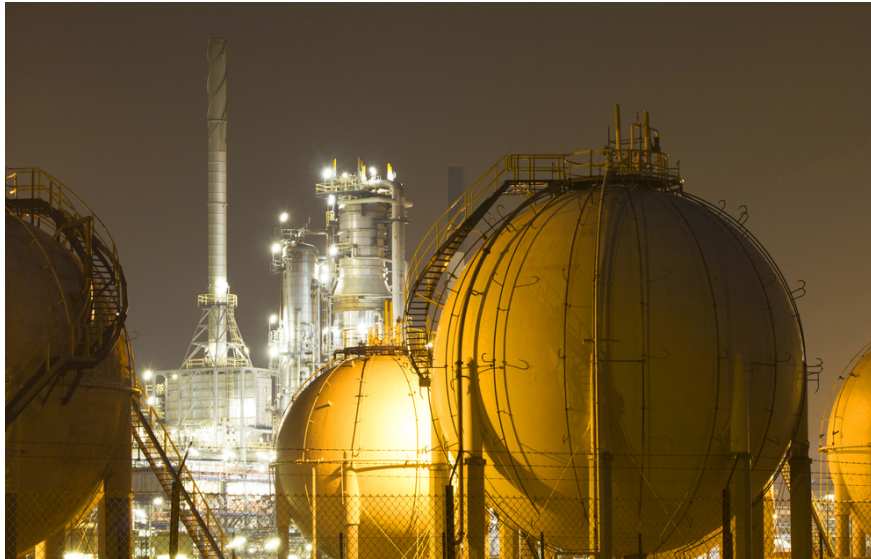
Gas storage tank
