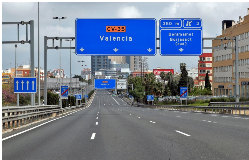
A view of the completely empty CV-35 road in Valencia, eastern Spain, 19 March, 2020
