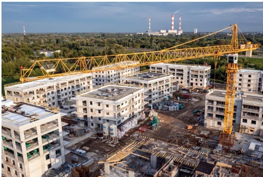
Construction in Warsaw, Poland
