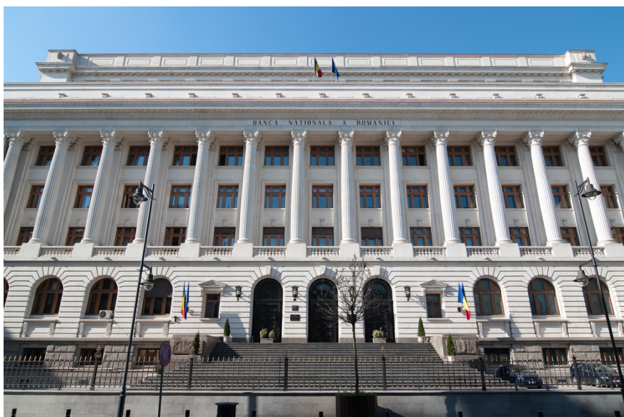
The National Bank of Romania building in Bucharest
