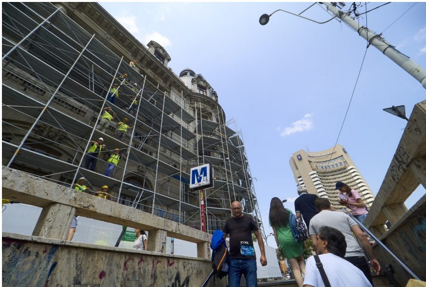
Restoration work on the Palace of the University of Bucharest
