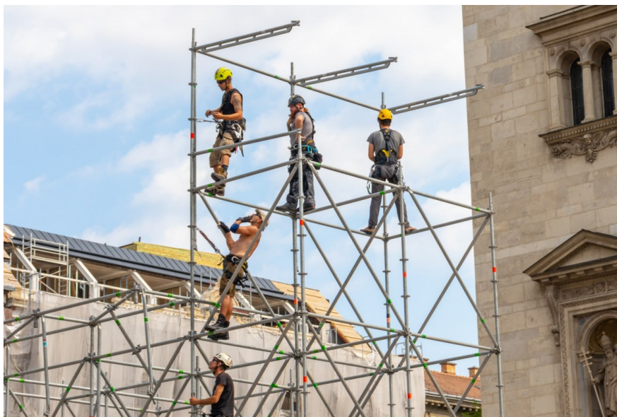
Construction workers in Budapest, Hungary
