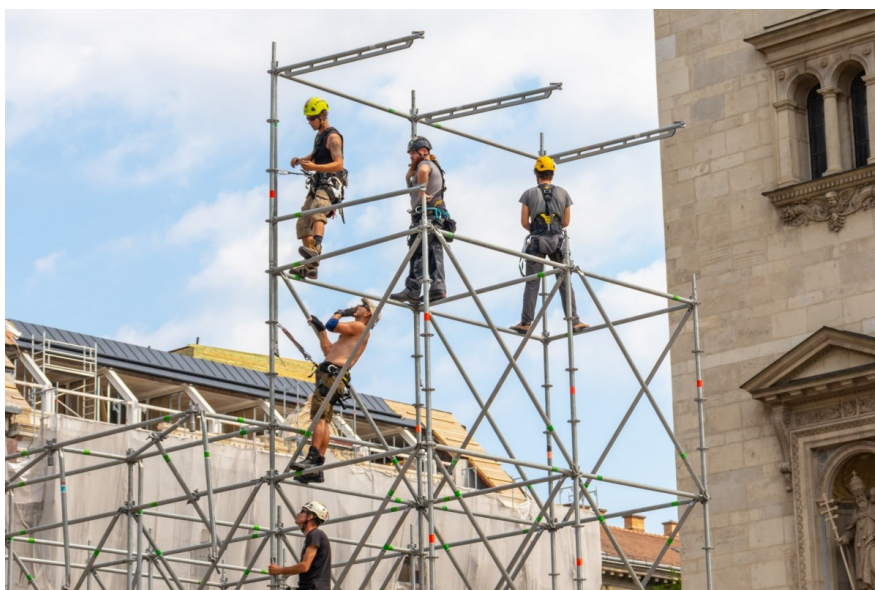
Construction workers in Budapest, Hungary
