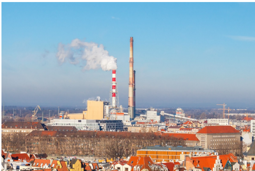
Thermal power plant in Wrocław, Poland
