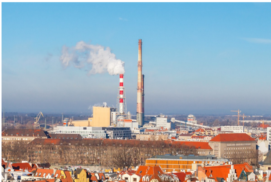
Thermal power plant in Wrocław, Poland
