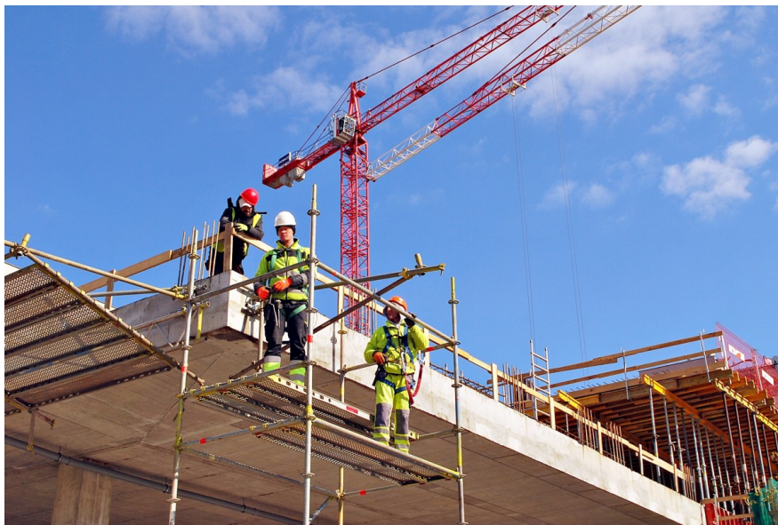
Construction workers in Warsaw, Poland
