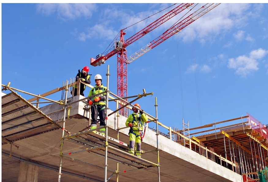
Construction workers in Warsaw, Poland
