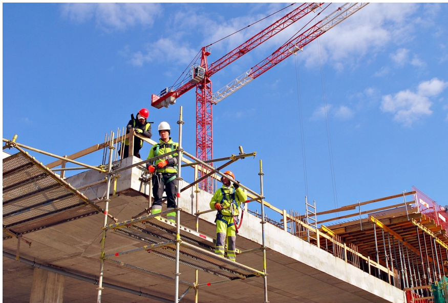
Construction workers in Warsaw, Poland
