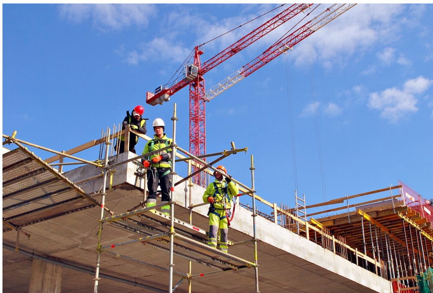
Construction workers in Warsaw, Poland
