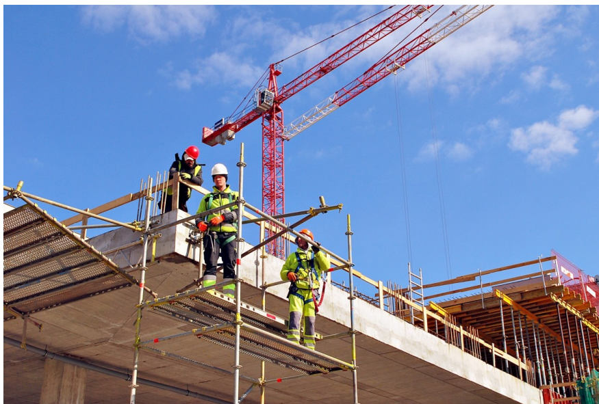
Construction workers in Warsaw, Poland
