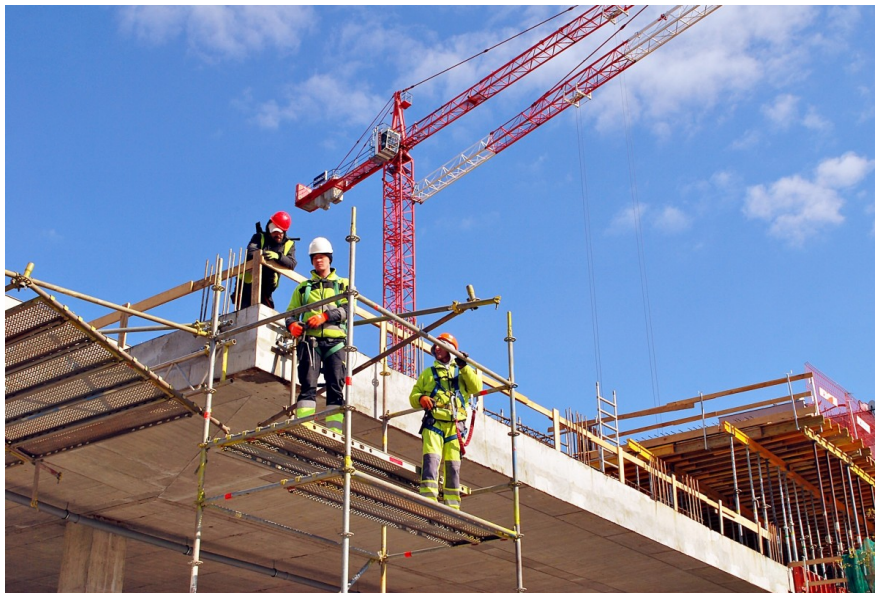
Construction workers in Warsaw, Poland
