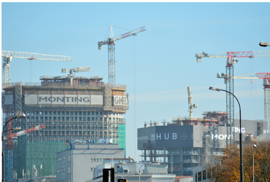
Construction of the 'Warsaw Hub', Poland
