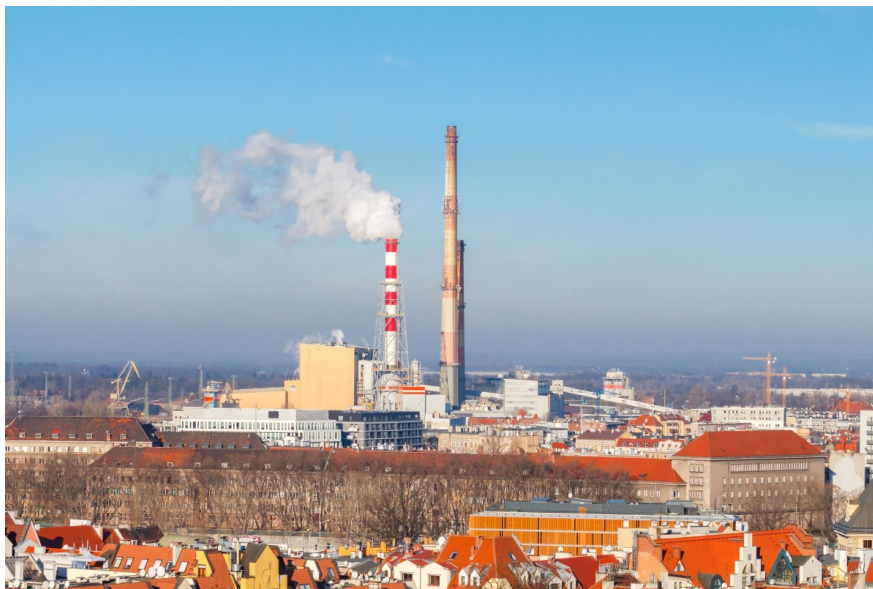
Thermal power plant in Wrocław, Poland
