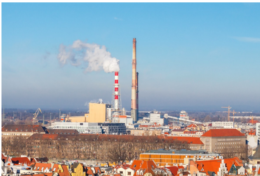
Thermal power plant in Wrocław, Poland
