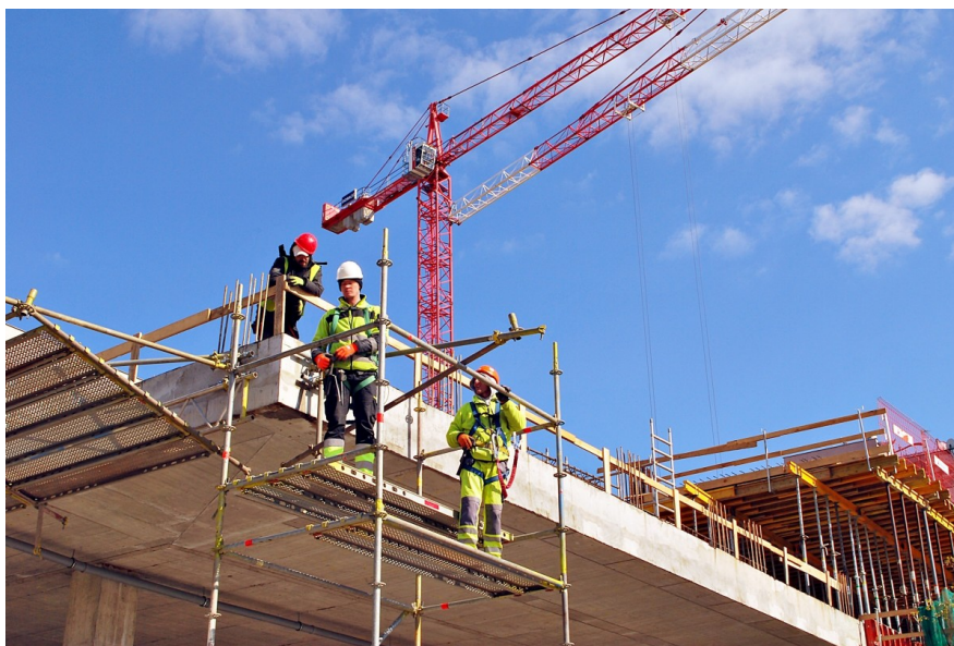
Construction workers in Warsaw, Poland
