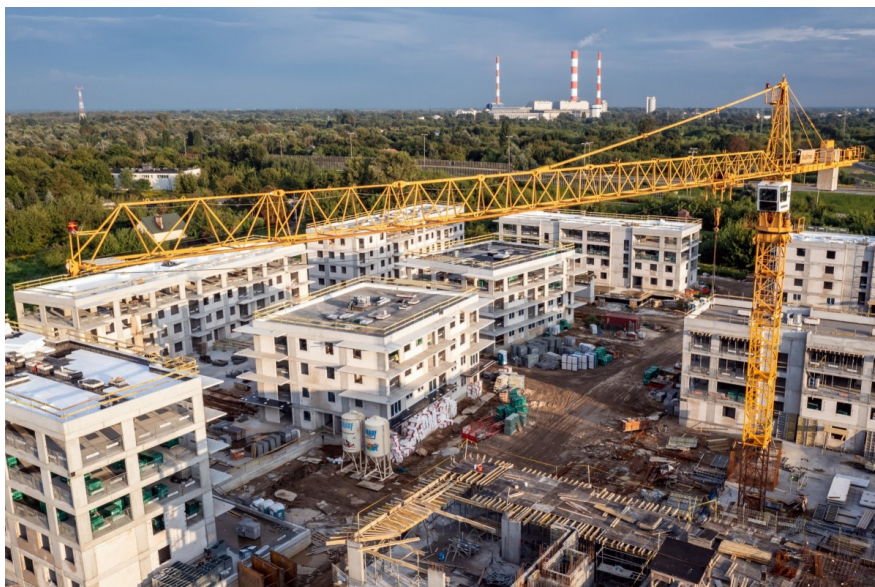
Construction in Warsaw, Poland
