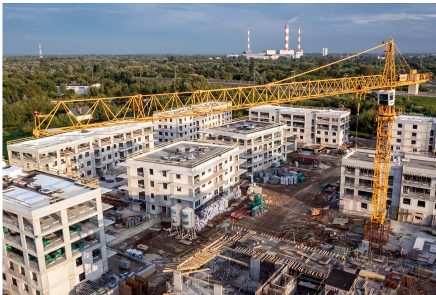
Construction in Warsaw, Poland
