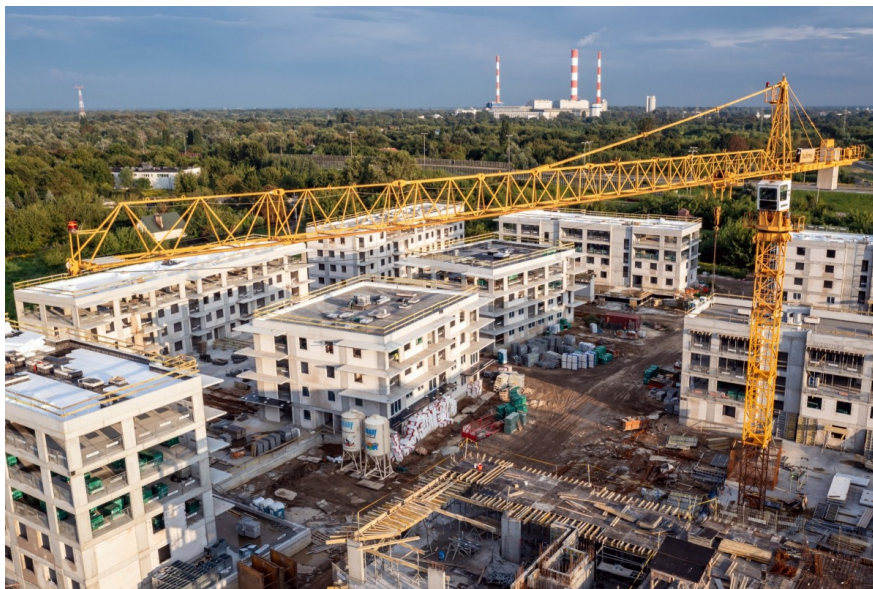
Construction in Warsaw, Poland
