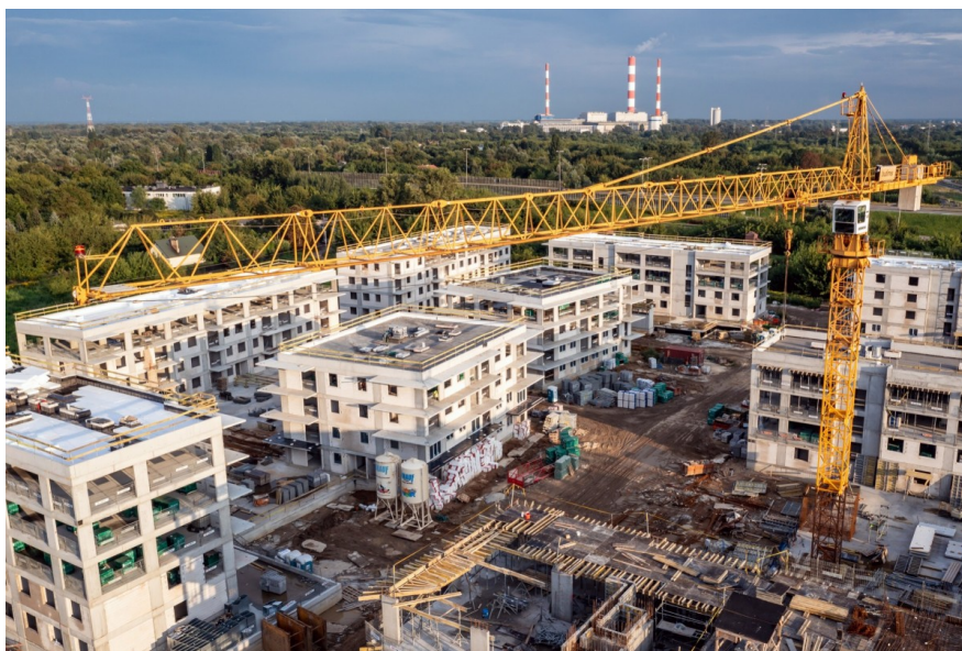
Construction output growth turned positive in Poland after 12 straight declines
