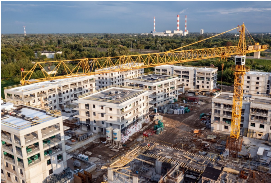
Construction in Warsaw, Poland
