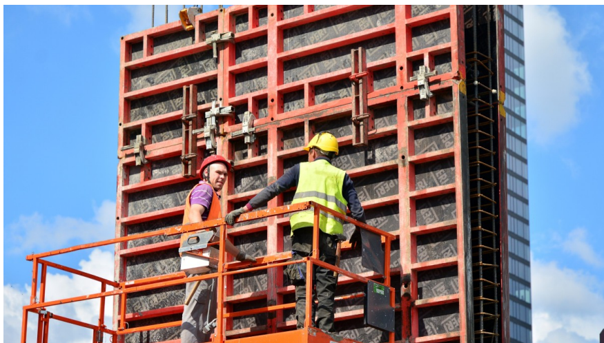
Polish workers at a construction site in Warsaw
