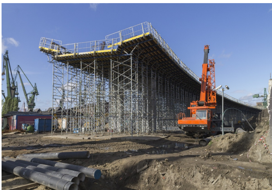
Construction of a bridge in Gdansk, Poland
