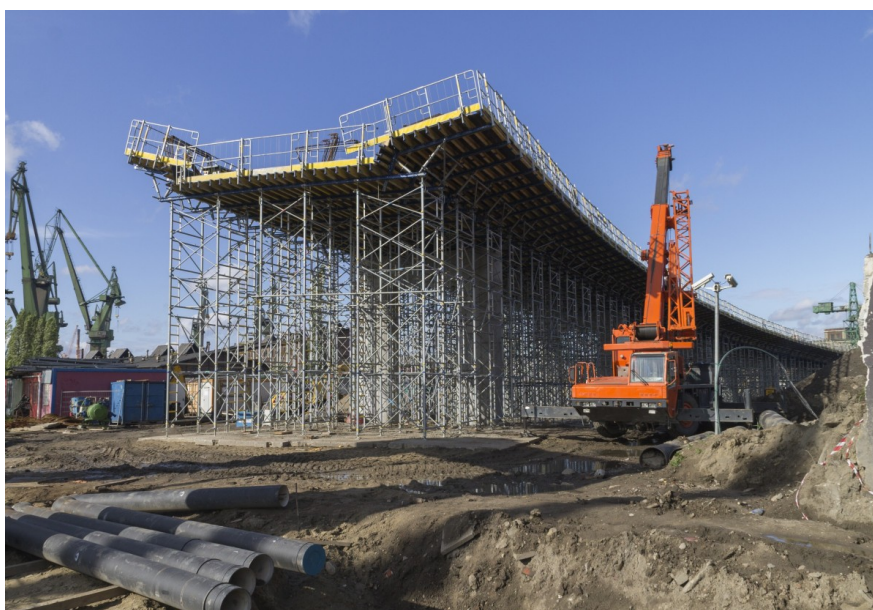
Construction of a bridge in Gdansk, Poland
