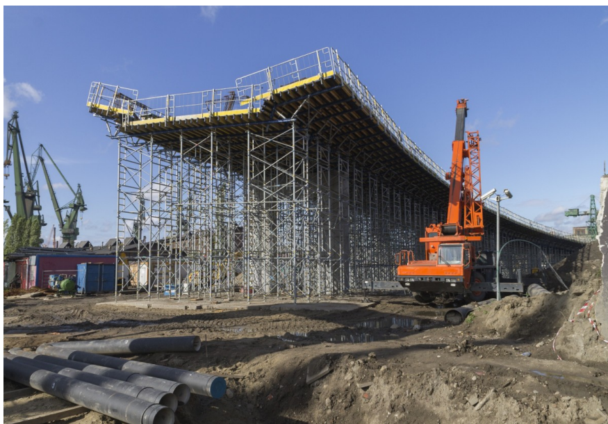
Construction of a bridge in Gdansk, Poland
