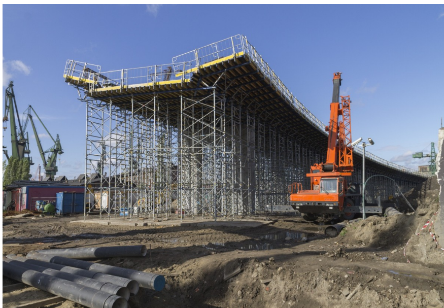
Construction of a bridge in Gdansk, Poland
