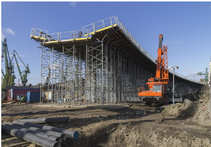
Construction of a bridge in Gdansk, Poland
