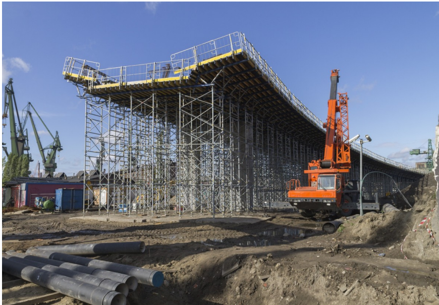
Construction of a bridge in Gdansk, Poland
