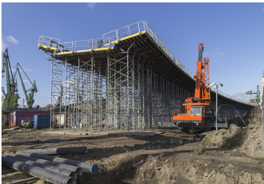
Construction of a bridge in Gdansk, Poland
