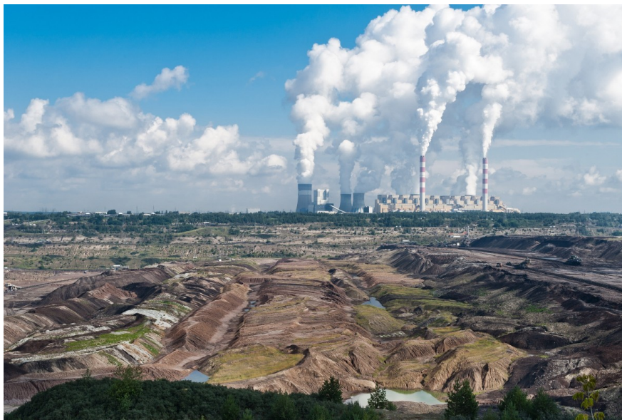
Coal power plant in Bełchatów, Poland
