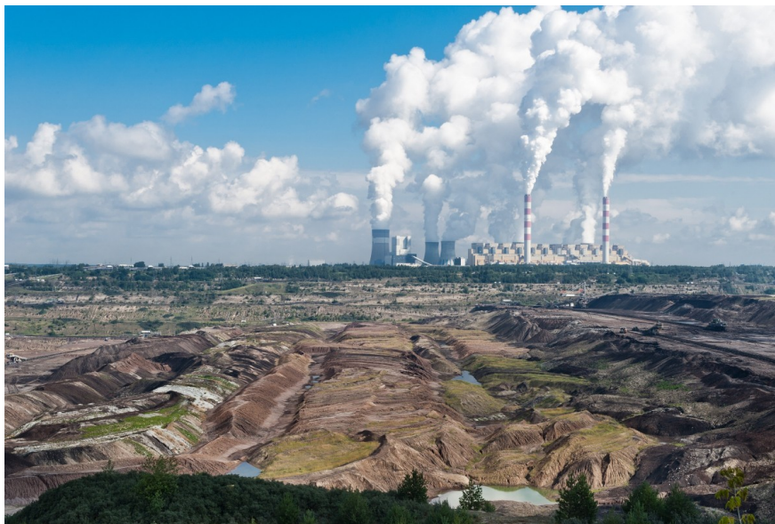
Coal power plant in Bełchatów, Poland
