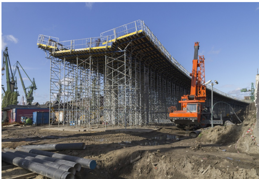
Construction of a bridge in Gdansk, Poland
