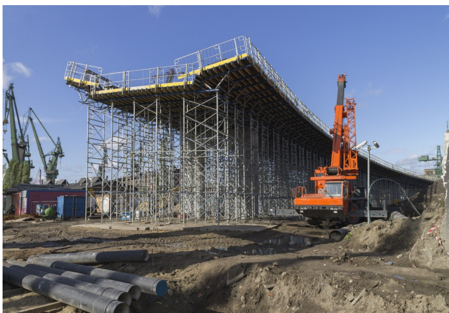
Construction of a bridge in Gdansk, Poland
