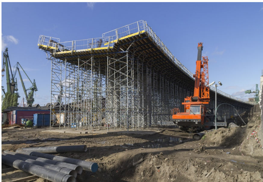
Construction of a bridge in Gdansk, Poland
