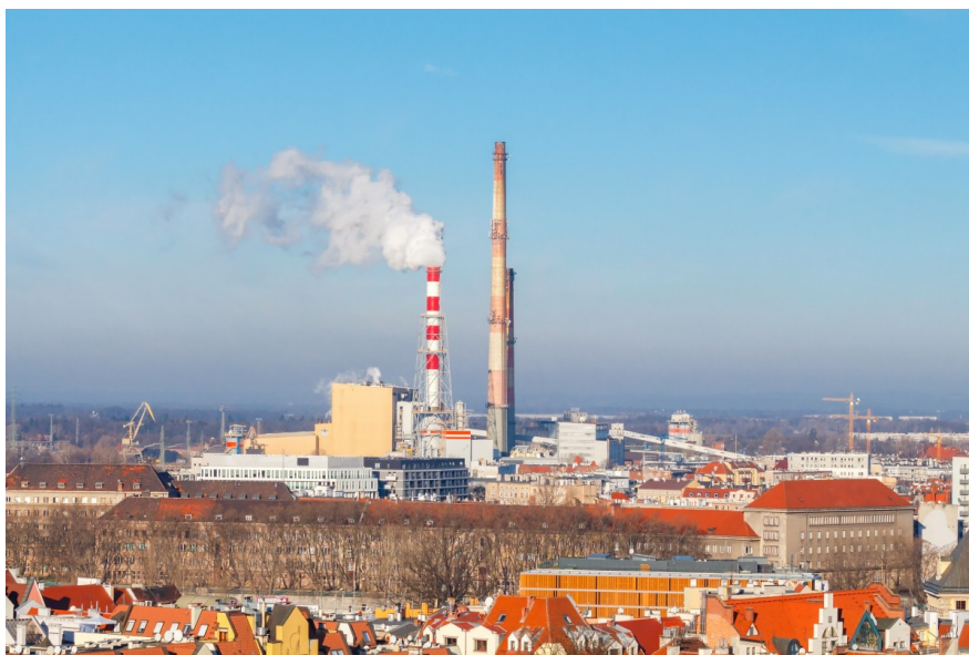
Thermal power plant in Wrocław, Poland
