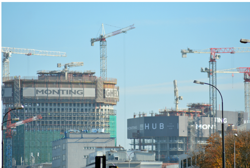
Construction of the 'Warsaw Hub', Poland
