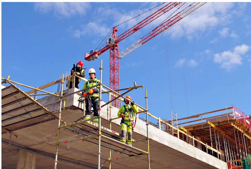
Construction workers in Warsaw, Poland
