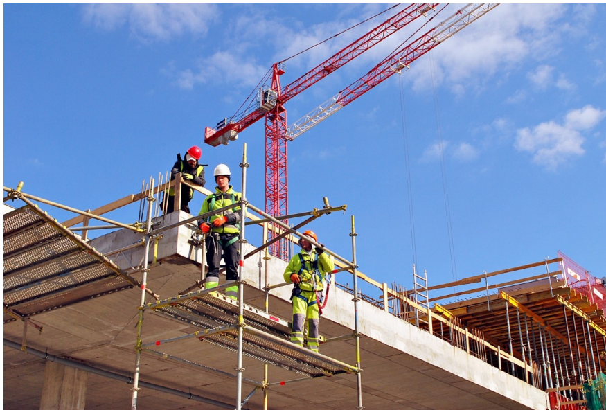
Construction workers in Warsaw, Poland
