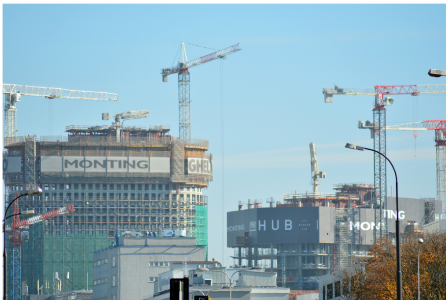
Construction of the 'Warsaw Hub', Poland
