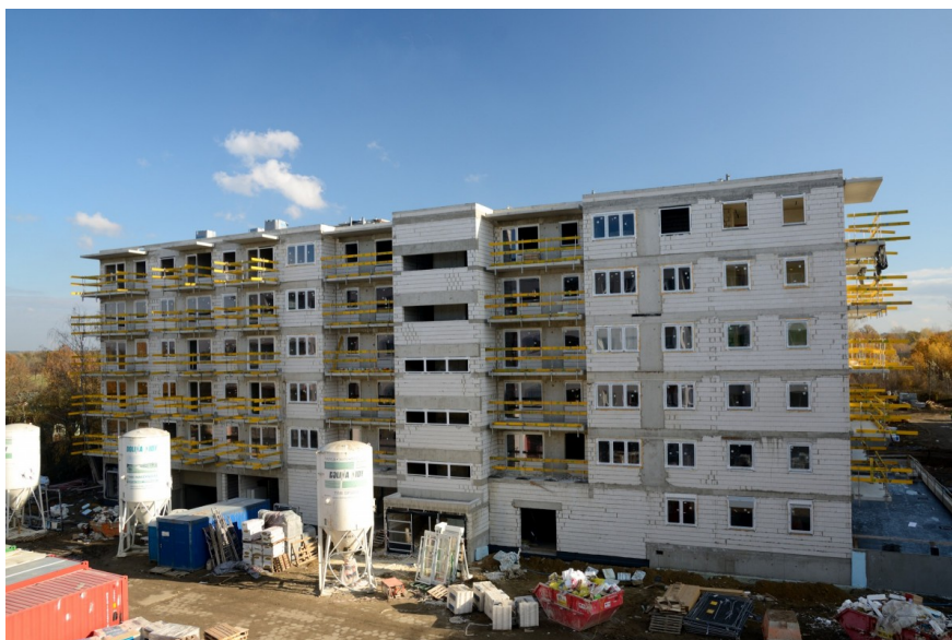
Another apartment building under construction in Warsaw
