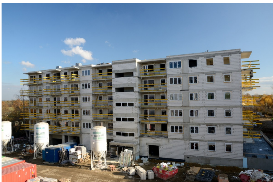
Another apartment building under construction in Warsaw
