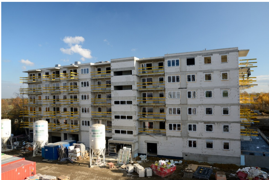
Another apartment building under construction in Warsaw
