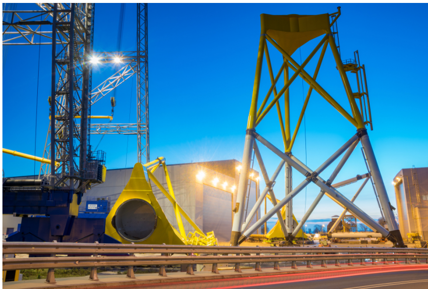
Wind power plant factory, Szczecin, Poland
