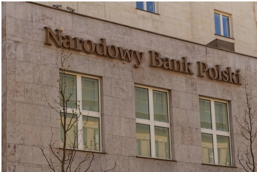
National Bank of Poland in Warsaw
