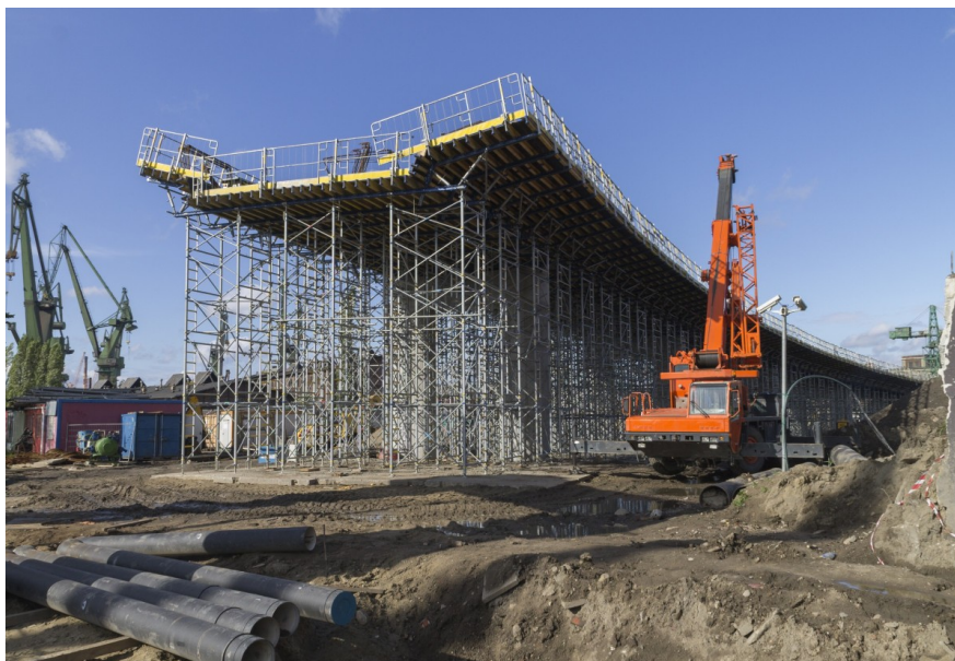
Construction of a bridge in Gdansk, Poland
