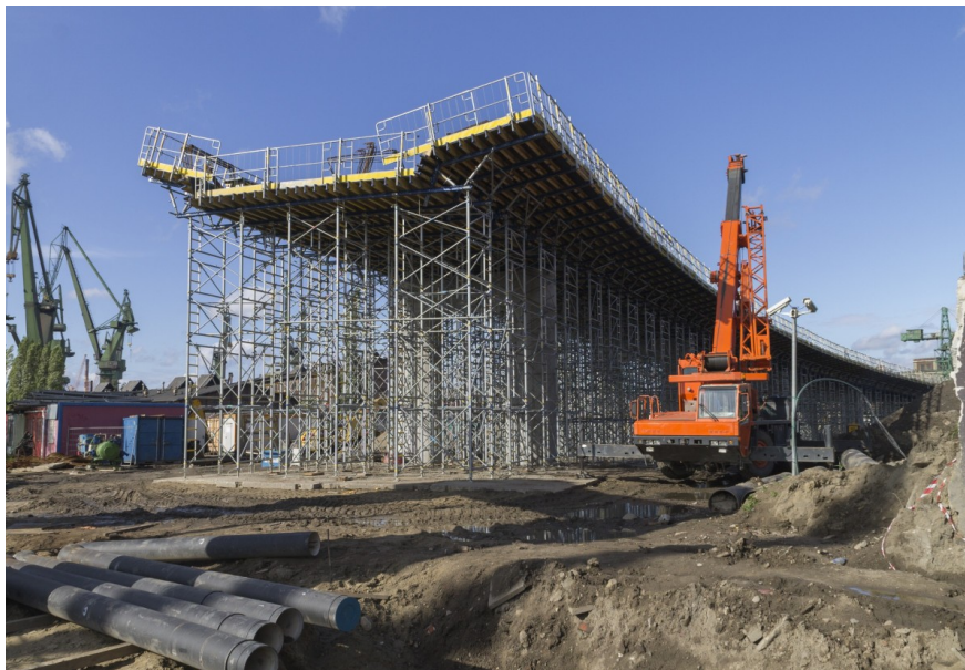
Construction of a bridge in Gdansk, Poland
