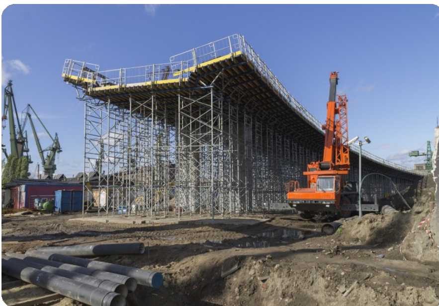
Construction of a bridge in Gdansk, Poland
