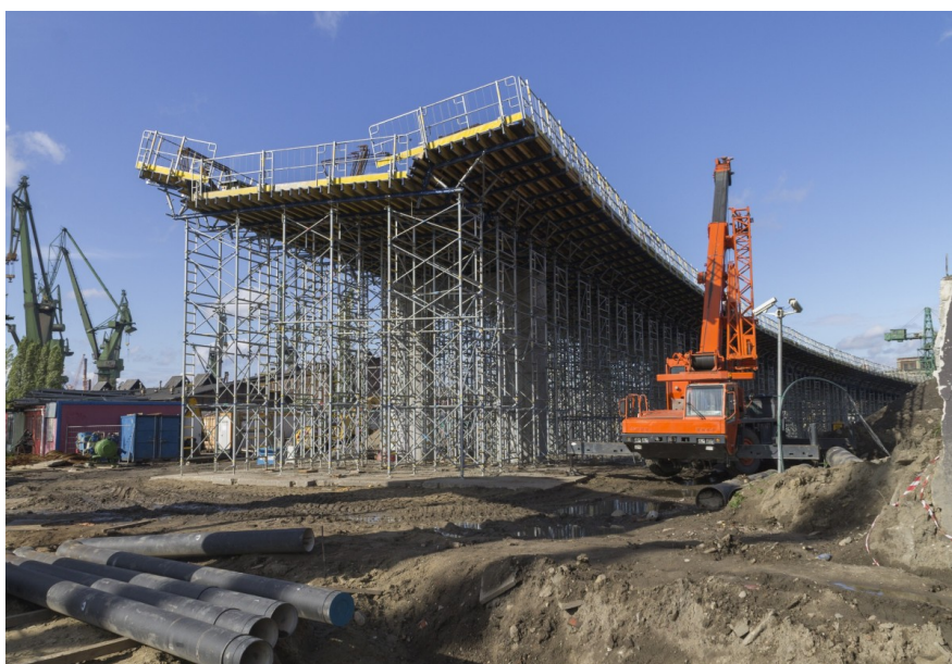
Construction of a bridge in Gdansk, Poland
