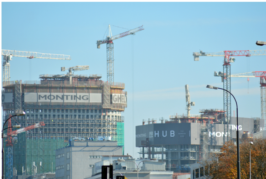
Construction of the 'Warsaw Hub', Poland
