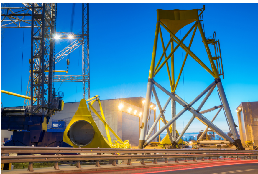
Wind power plant factory, Szczecin, Poland
