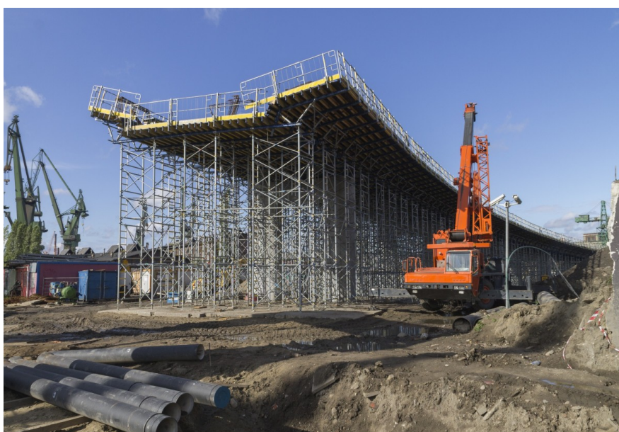
Construction of a bridge in Gdansk, Poland
