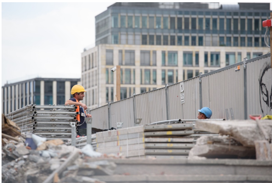
Construction work in Warsaw, Poland
