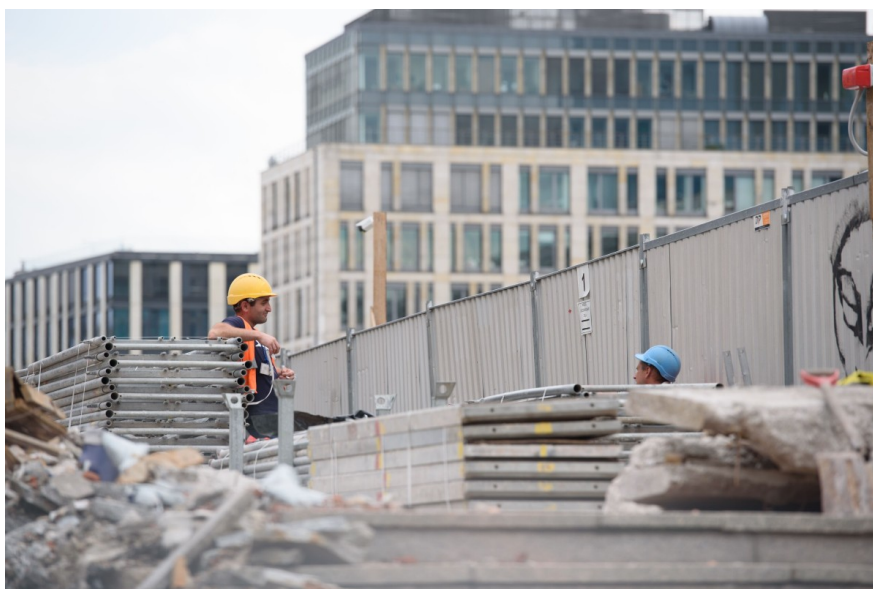
Construction work in Warsaw, Poland
