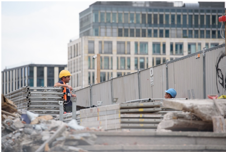
Construction work in Warsaw, Poland
