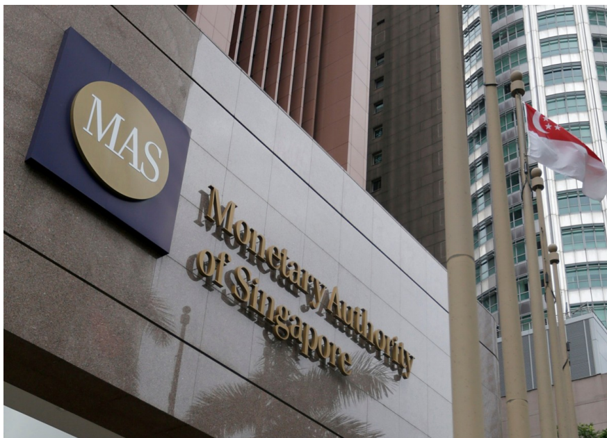
View of the Monetary Authority of Singapore (MAS) building in Singapore
