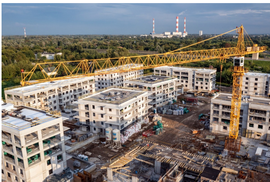
Construction in Warsaw, Poland
