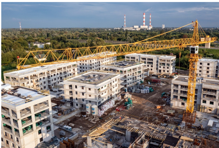
Construction in Warsaw, Poland
