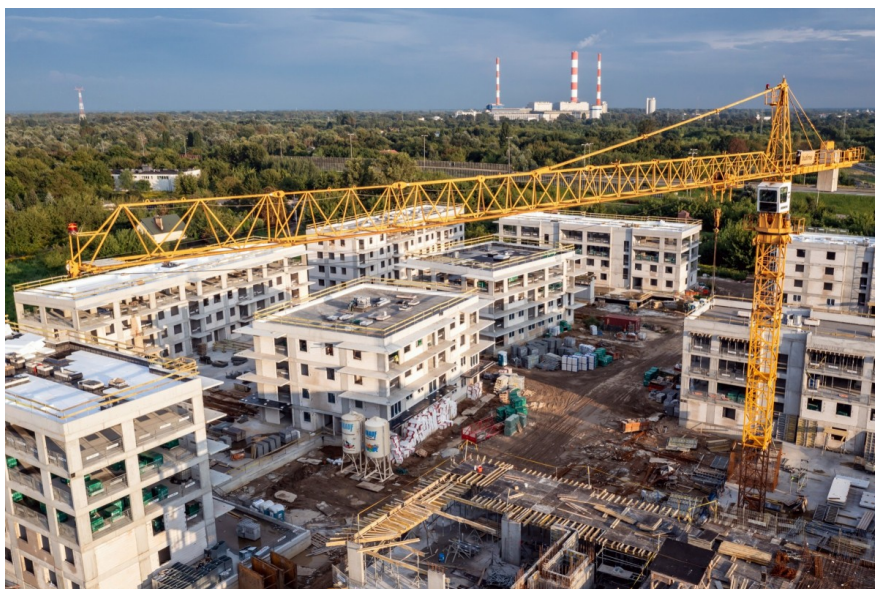
Construction in Warsaw, Poland
