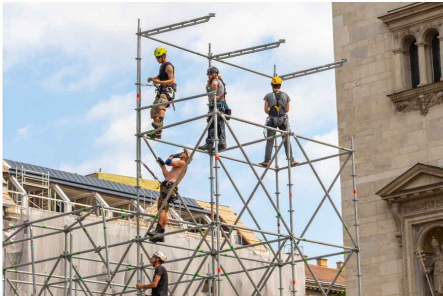
Construction workers in Budapest, Hungary
