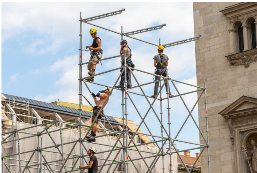
Construction workers in Budapest, Hungary
