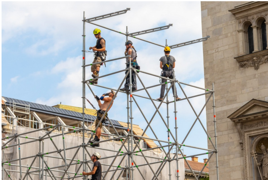
Construction workers in Budapest, Hungary
