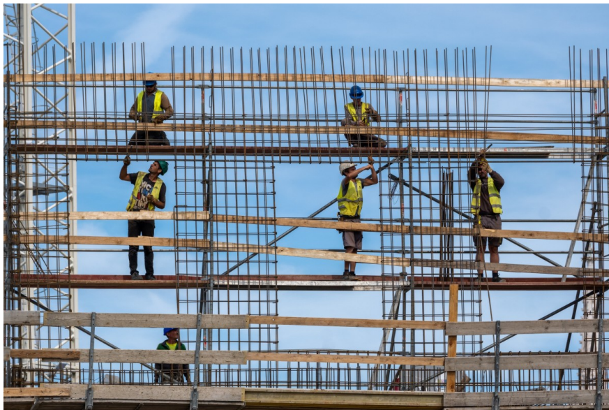
Workers at a construction site in Budapest, Hungary
