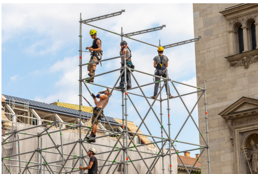
Construction workers in Budapest, Hungary
